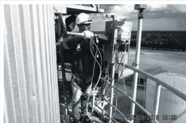
Accuracy verification of Continuous Emission Monitoring Systems (CEMs)
