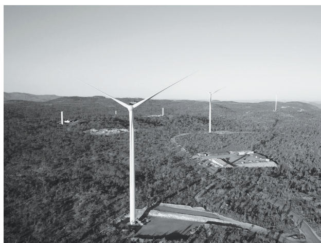
180.45-MW Mount Emerald Wind Farm, Victoria, Australia
